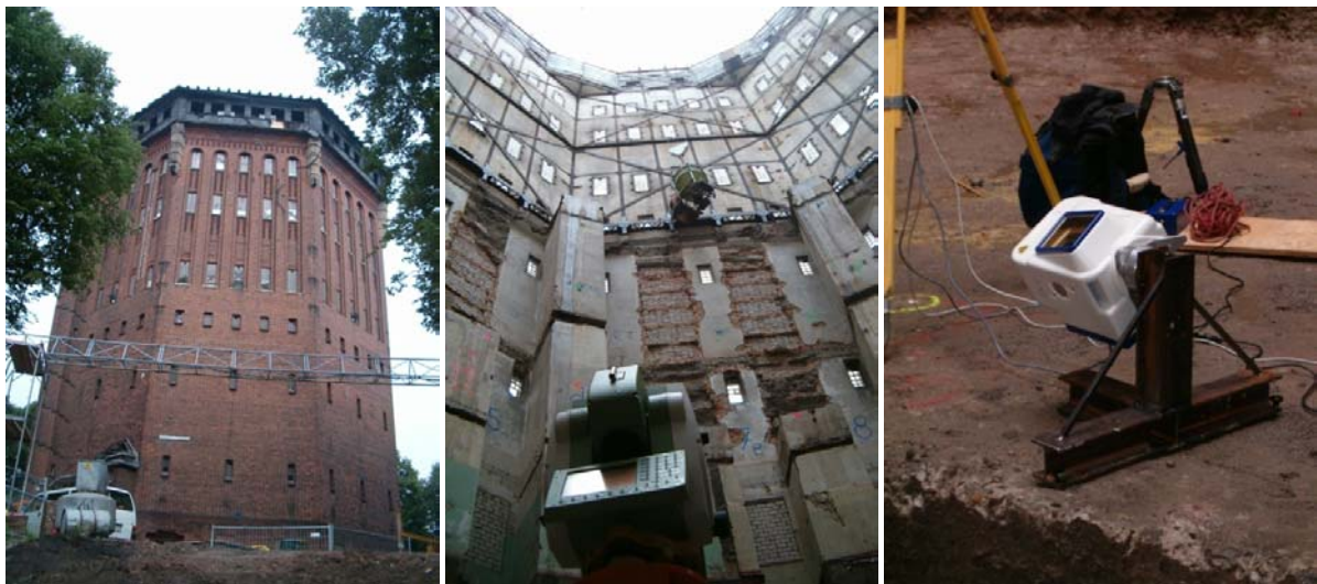
Figure 2: Former water tower at Sternschanzen Park in Hamburg: view at the external facade (left), interior view (centre), scanner GS100 on the special socket on the ground level of the tower (right)
