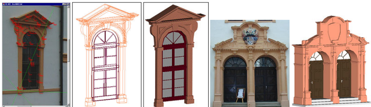
Fig. 6: Measurement, reconstruction and rendering of a window of Celle castle (from left to right), ornate doorway as a photo and as a generalized reconstructed doorway (right)
