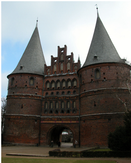
Figure 2. Western facade front of the Holstentor, Lübeck
